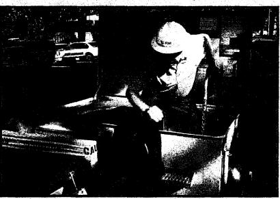
Ground Access Points usually are reserved for accessing underground vaults at large Controlled Environment Vault (CEV) installations (this one houses equipment that can deliver telephone and broadband service to multiple neighborhoods).
